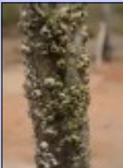
Barnacle fouling (below) and mussel fouling (above) on wooden structures.
