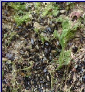
Barnacle fouling (below) and mussel fouling (above) on wooden structures.
